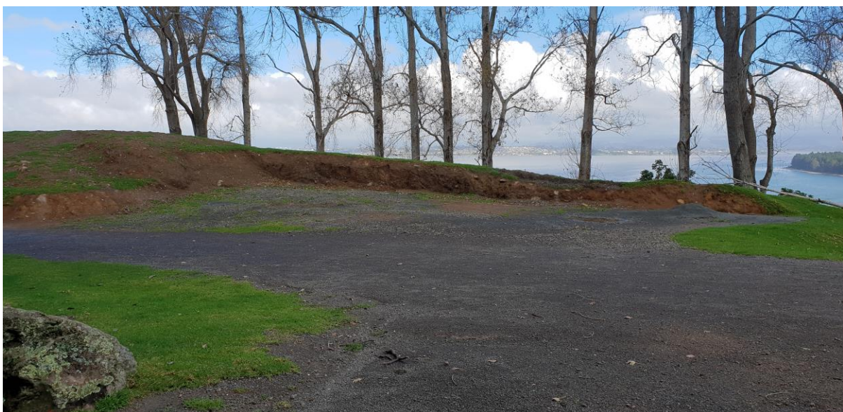
Figure 3: Slip debris spoil stock pile after restacking and shaping (InSitu Heritage Ltd April 2018).
